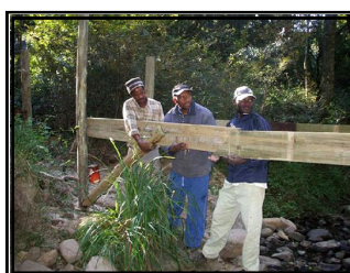
Tom Dyantjies and helpers making the frame for the bridge.
