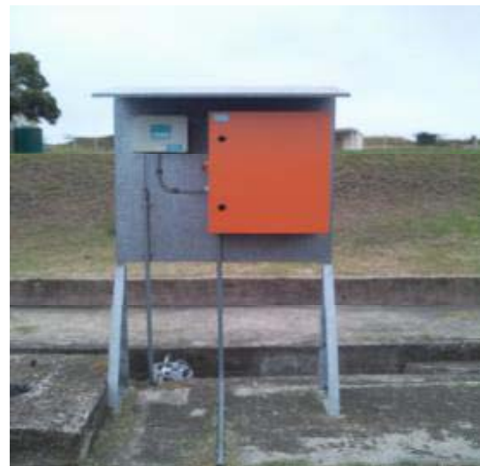
New Flow Meter installed
